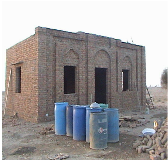
Under construction Mosque for Bado Jabal Villagers
