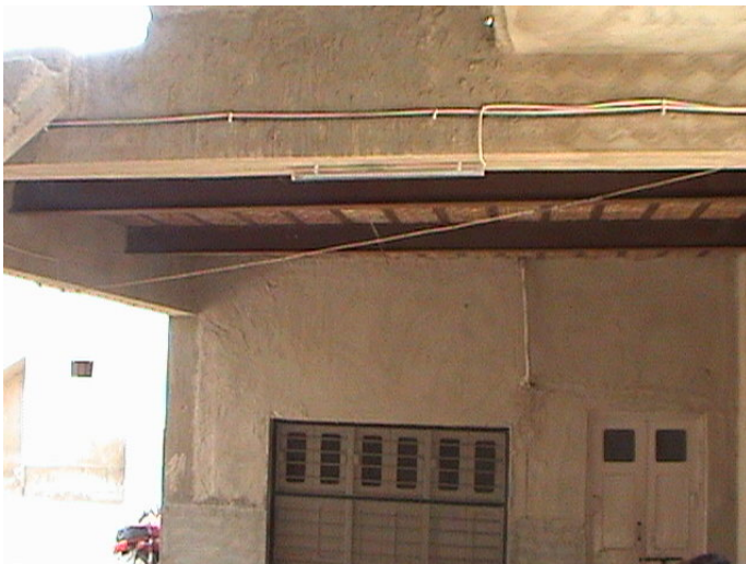
Solar power LED based light installed at Dr. Mehdi's house
